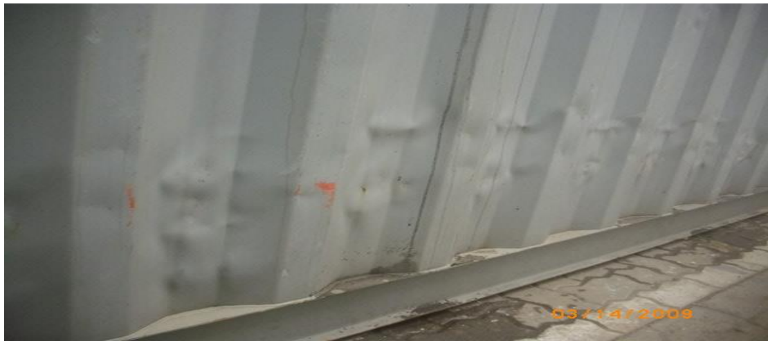
4. Old repairs on panels (straightening)
