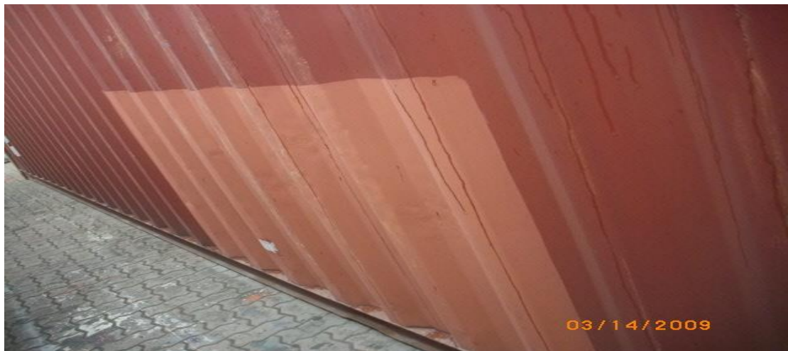
5. Old repairs on panels (straightening)
