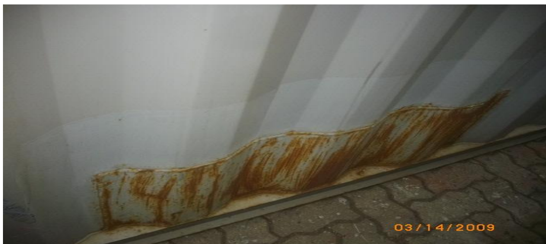
3. Old repairs on panels (patches, inserts, etc.)
